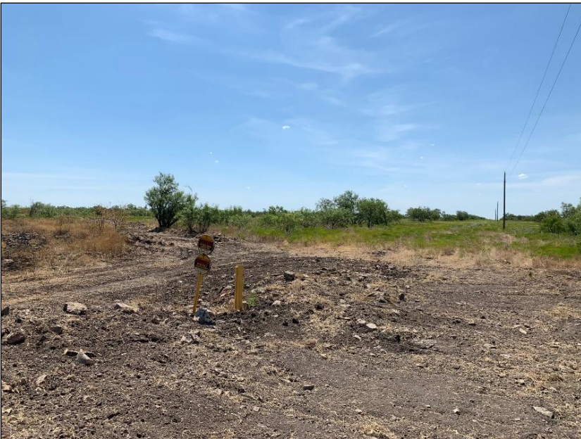
Dozer line across the first of three pipelines
