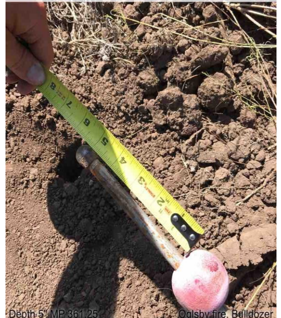
Depth gauge showing approx. 5" from dozer line to pipeline
